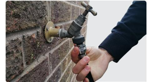
2. Connect the **RED** hose from the waste water outlet and direct to a drain or nearby soakaway
